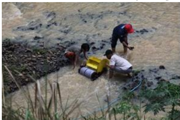
Figure 6. The spiral Archimedes pump installed in Plana River close to the pump with solar panel.
