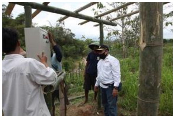
Figure 7. Installation of solar water pump.
