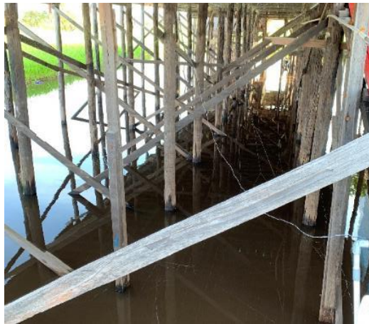
Figure 7. Signs that the water is starting to recede.
