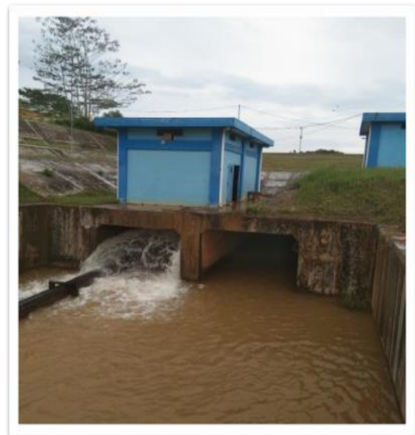
Figure 2. Balikpapan Teritip Dam
