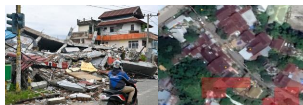
Figure 15. Damage Detected at Residents' Houses
