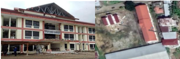
Figure 17. No Damage Detected at Mamuju Police Dormitory
