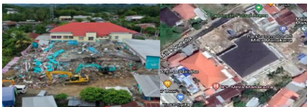
Figure 18. No Damage Detected at Mitra Manakarra Hospital
