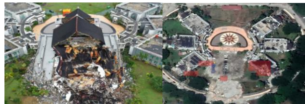
Figure 11. Damage Detected at Governor's Office
